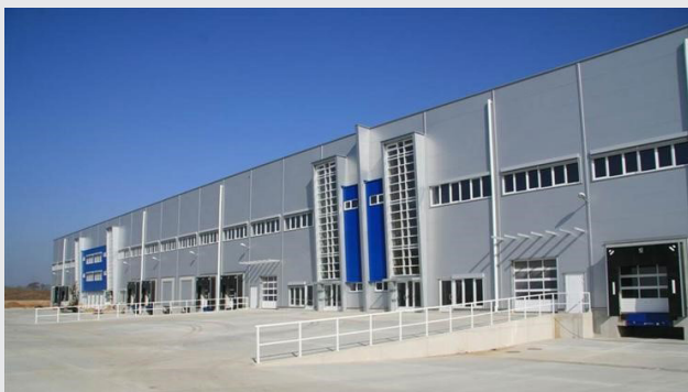
Logistics center Hagenbrunn
